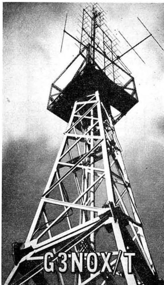
A view of the aerial mast at G3NOX/T. The working platform is at the 28 ft. level. Since this picture was taken, the tower has been extended to 40 ft.
